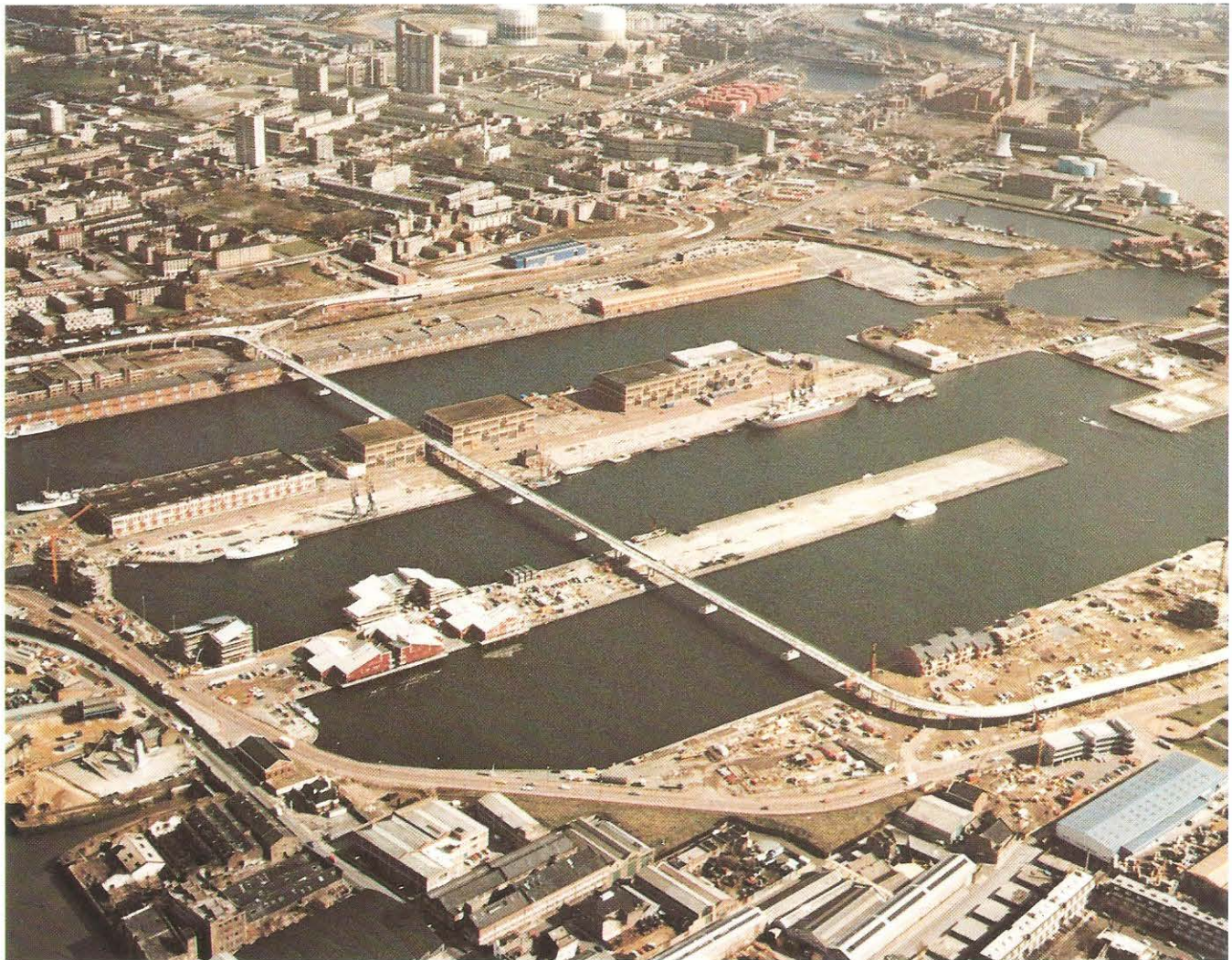
Aerial view showing the Docklands Light Railway crossing the West India Docks with the Delta Junction and the Operations and Maintenance Centre at the top of the picture.
