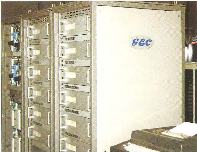
SSI (solid state interlocking) cubicles and line printer.
