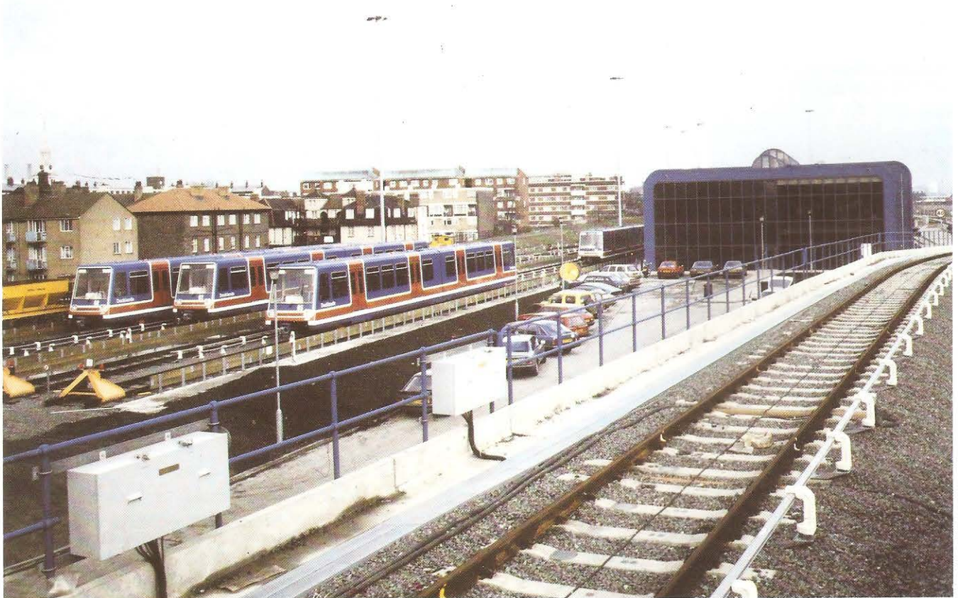
The Operations and Maintenance Centre (OMC) and stabling sidings as seen from Poplar Station.
